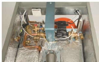
Flow, return, hot and cold valve connections
